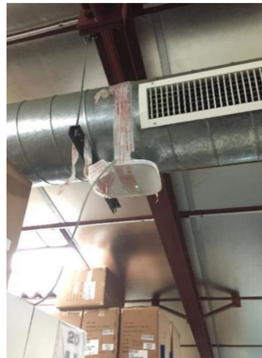
Duct Tape on a Duct
